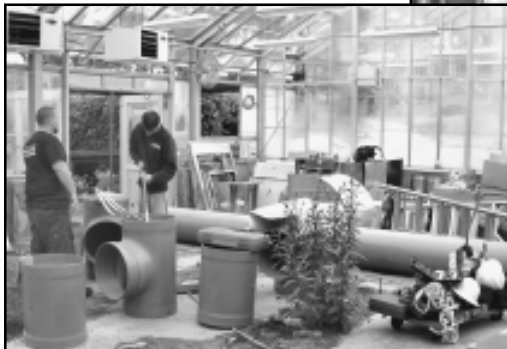
OH Greenhouse renovations.
